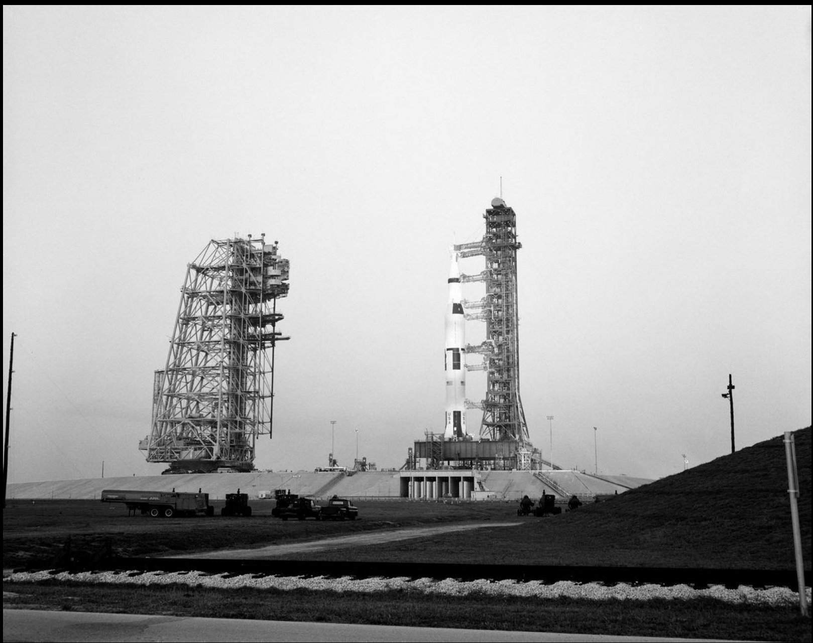
Arming Tower – Mobile Service Structure
